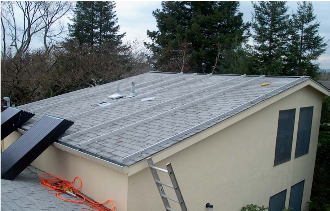
Mounting rails are installed and awaiting the panels.
