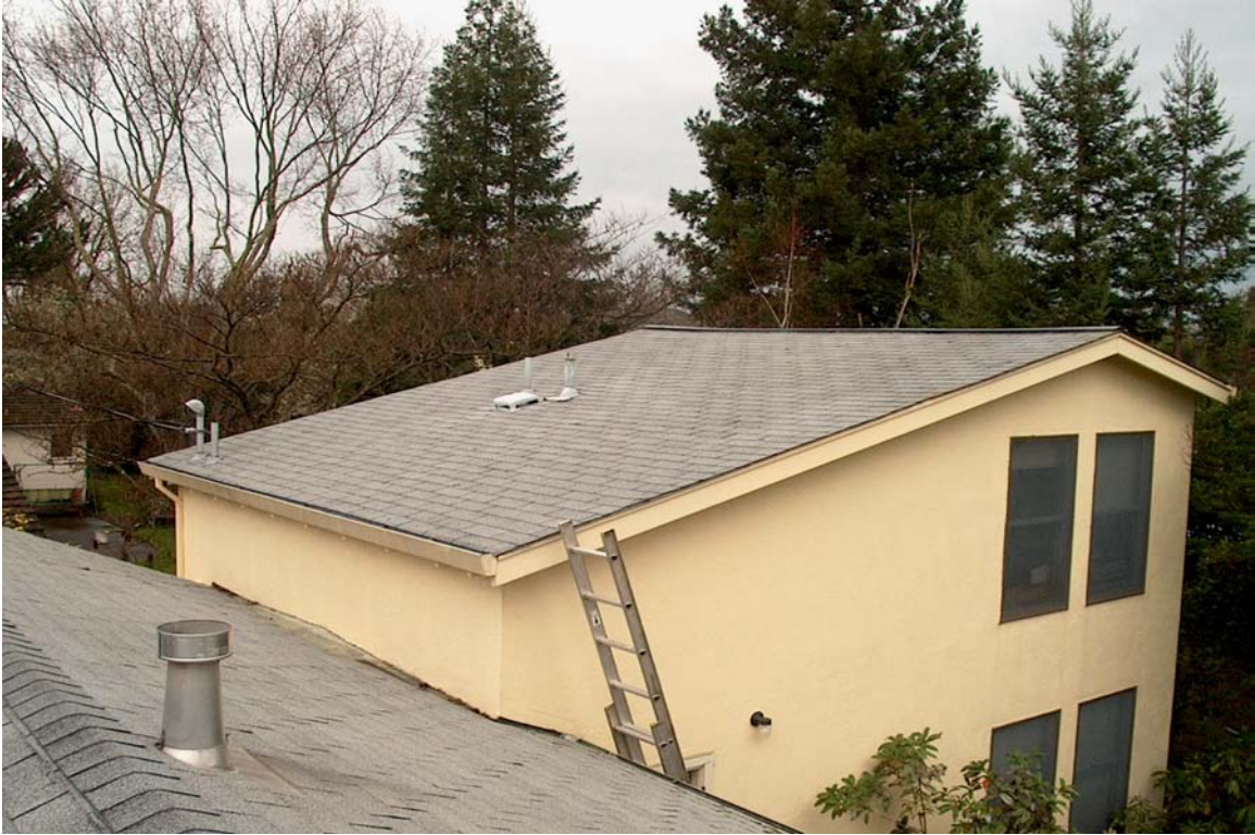
With the tree gone, the roof is ready for panel installation.
